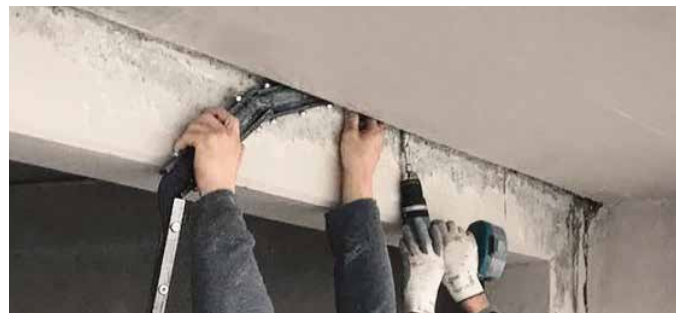
DESOI Quick Seal - Montage | DESOI Quick Seal - installation
